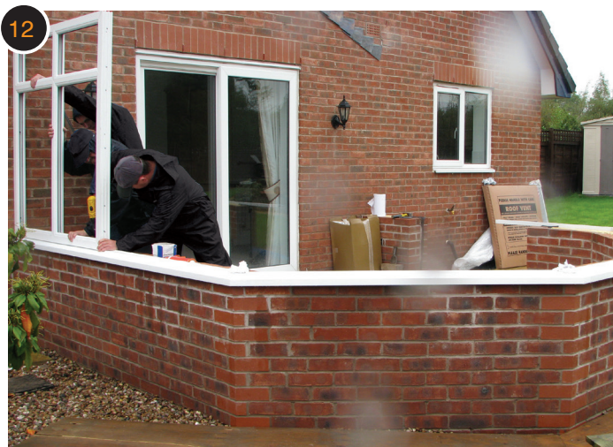
The PVCu external cill is fitted to the dwarf wall and the erection of the side frames begins.
