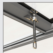
Pole operated screw jack mechanism
