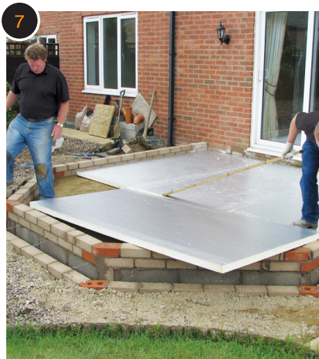
Floor insulation and a damp proof membrane are laid over the sand.
