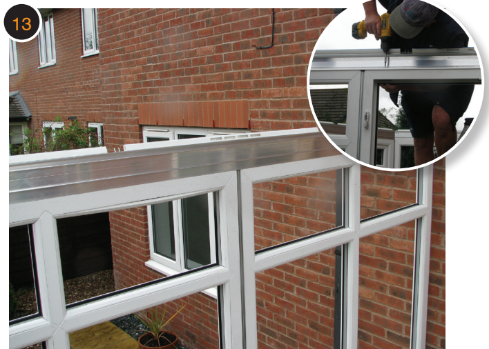
On completion of the frames a structural aluminium eaves beam is fitted to the head of the frames.
