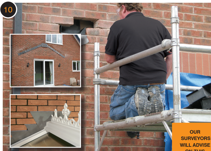
Cavity trays may be installed depending on the porosity of the house masonry. Otherwise a standard flashing is used.
