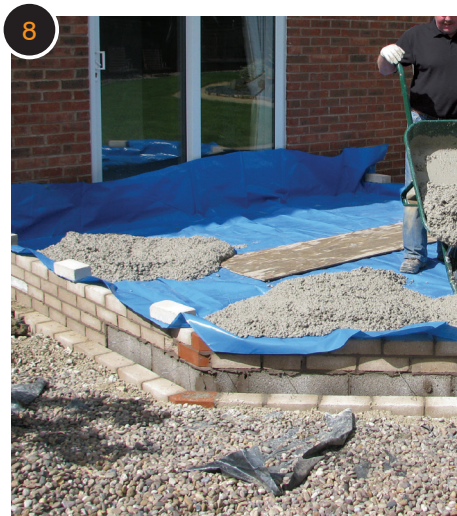
Concrete 100mm thick is laid to bring the slab up to the finished floor level.
