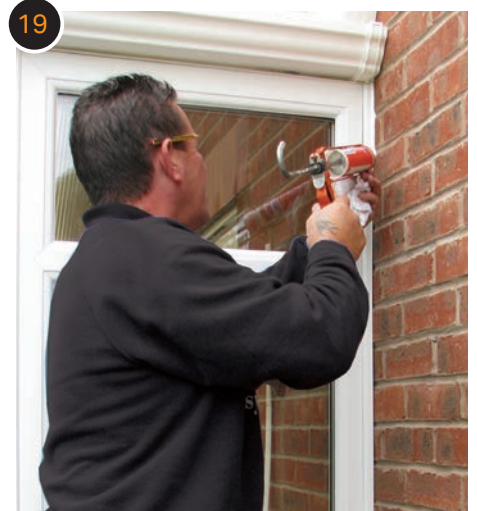
All the finishing touches are added to the conservatory, including the sealing of the side frames against the house wall.
