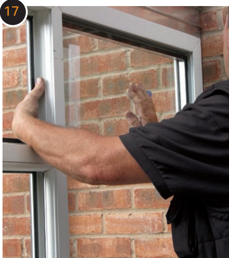
The glazing is installed into the side frames.
