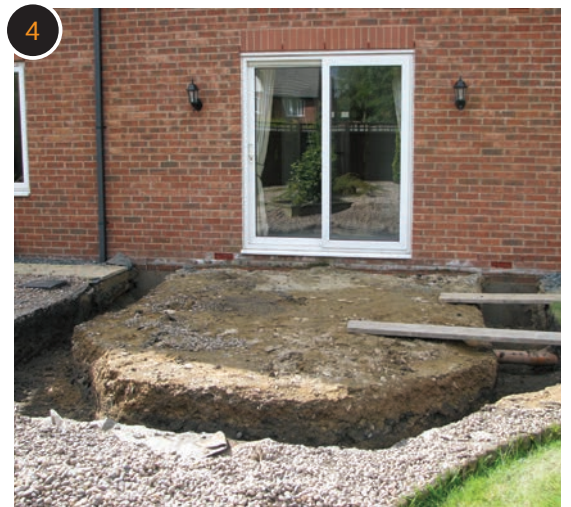
Footings are dug to a minimum depth of 450mm - this will vary depending on the ground conditions.
