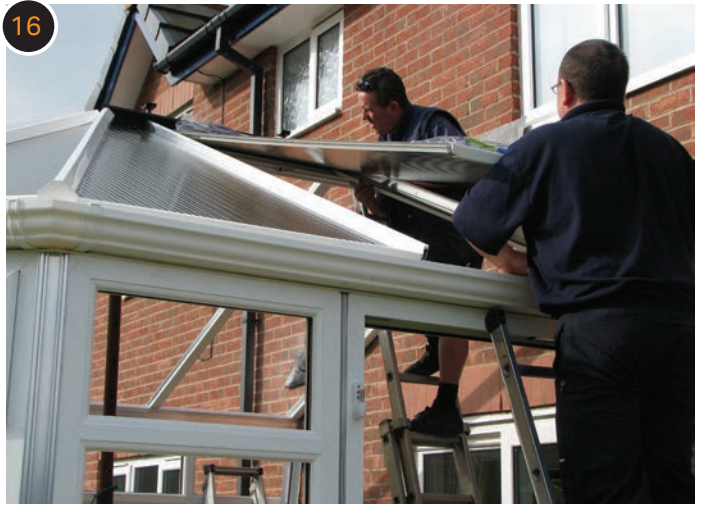
The chosen glazing panels or sealed units are installed.
