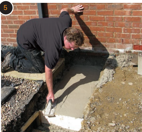
The concrete is floated to form a level surface area to build upon.
