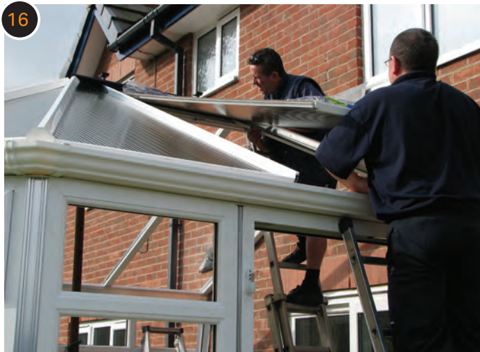
The chosen glazing panels or sealed units are installed.
