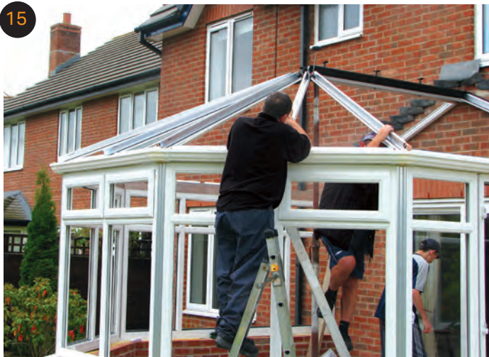
Now the roof is built - the glazing bars are fixed from the eaves beam to the ridge.
