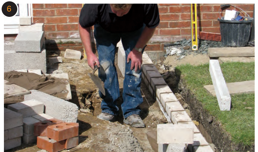
The outer leaf of the cavity wall is built to just below outside ground level.
