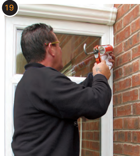
All the finishing touches are added to the conservatory, including the sealing of the side frames against the house wall.
