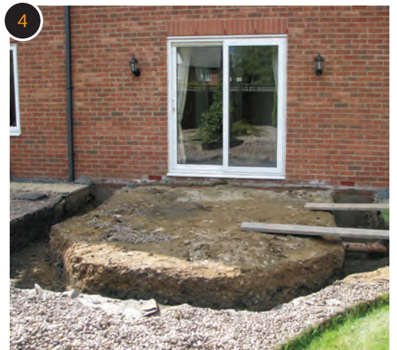
Footings are dug to a minimum depth of 450mm - this will vary depending on the ground conditions.
