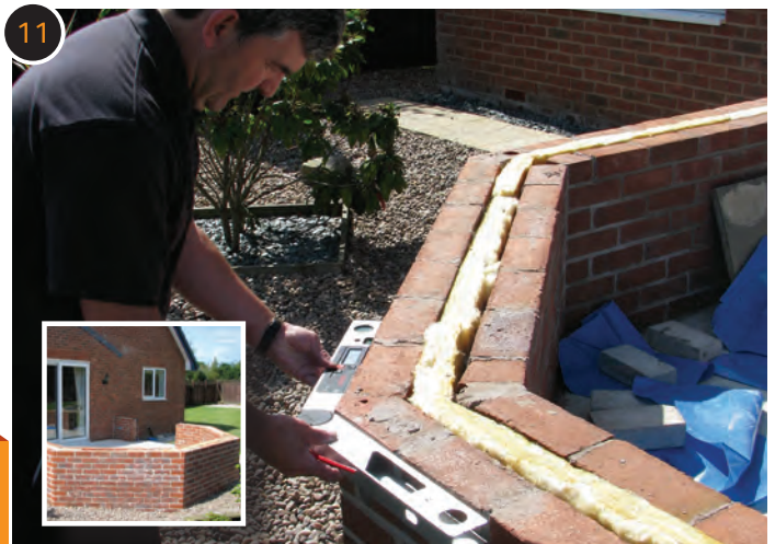
The dwarf walls are built to the height agreed and will include insulation in the cavity wall.
